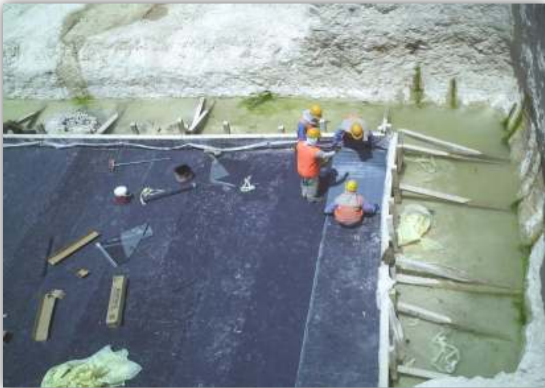
CP 361/3a North sewer rising main Water Proofing Membrane Laying
