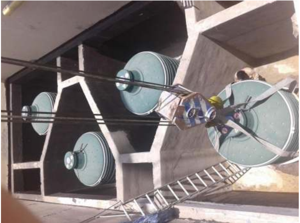
HILTON HOTEL TANK ROOM CONSTRUCTION AND NEW GAS TANKS
