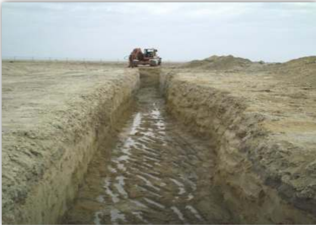
QD/TAC/C/2005- 2006/004/sub-44 visitor's road 1000mmØ GRP Pipe Excavation
