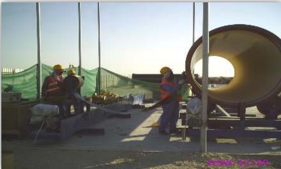
CP 361/3A North Sewer Rising Main (1600mm Dia Pipe Wrapping)
