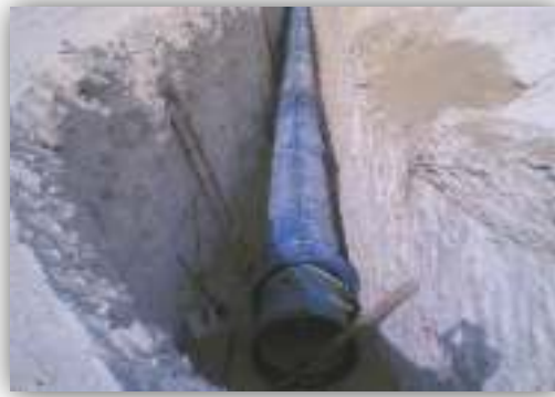
QD/TAC/C/2005- 2006/004/sub-44 Visitor's Road 700mm Dia GRP Pipe Laying
