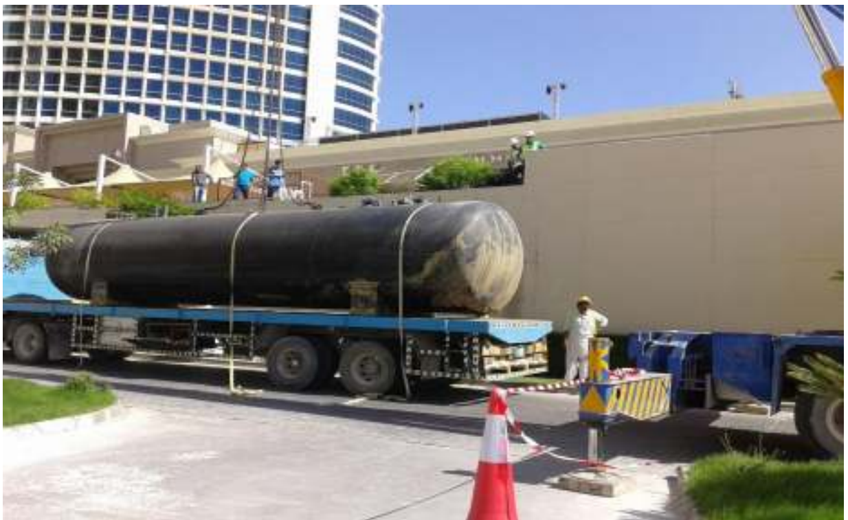
HILTON HOTEL REMOVAL OF OLD GAS TANK
