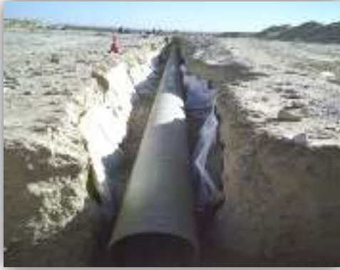
QD/TAC/C/2005- 2006/004/sub-44 Visitor's Road 700mm Dia GRP Pipe Laying
