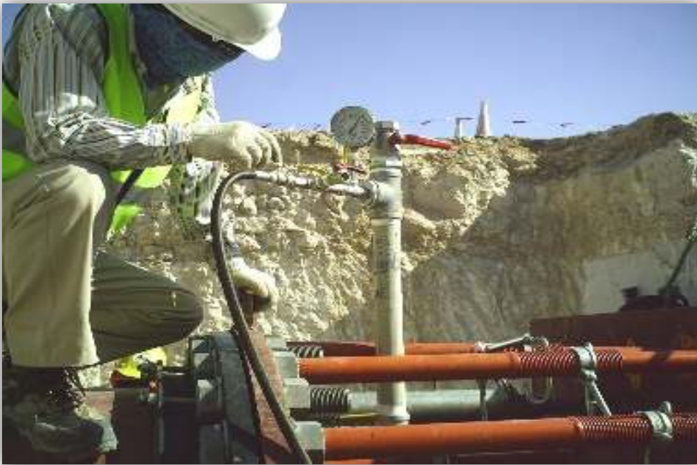
CP 361/3A North Sewer Rising Main (1600mm Dia Pipe Testing)
