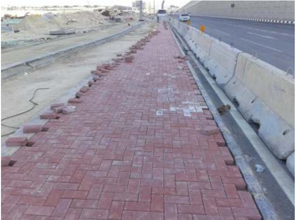
INTERLOCK PAVING WORKS AT EAST INDUSTRIAL ROAD
